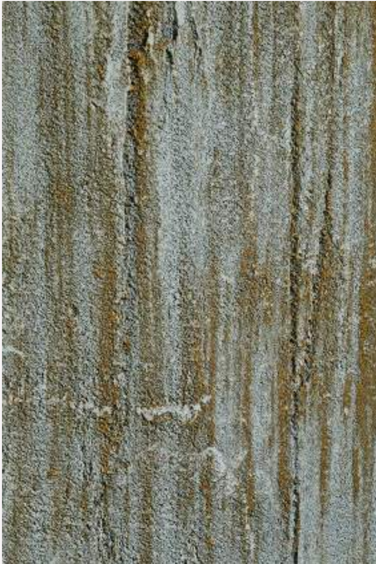
CONCRETE BY NOVACOLOR 17008 & IRONIC & FASE SILOSSANICA 6101
